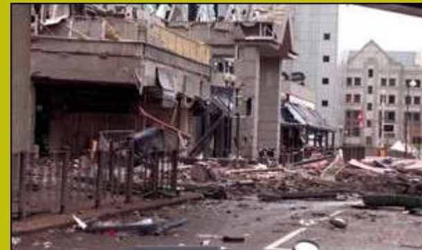
Radiocommunications Agency Building, 1996
